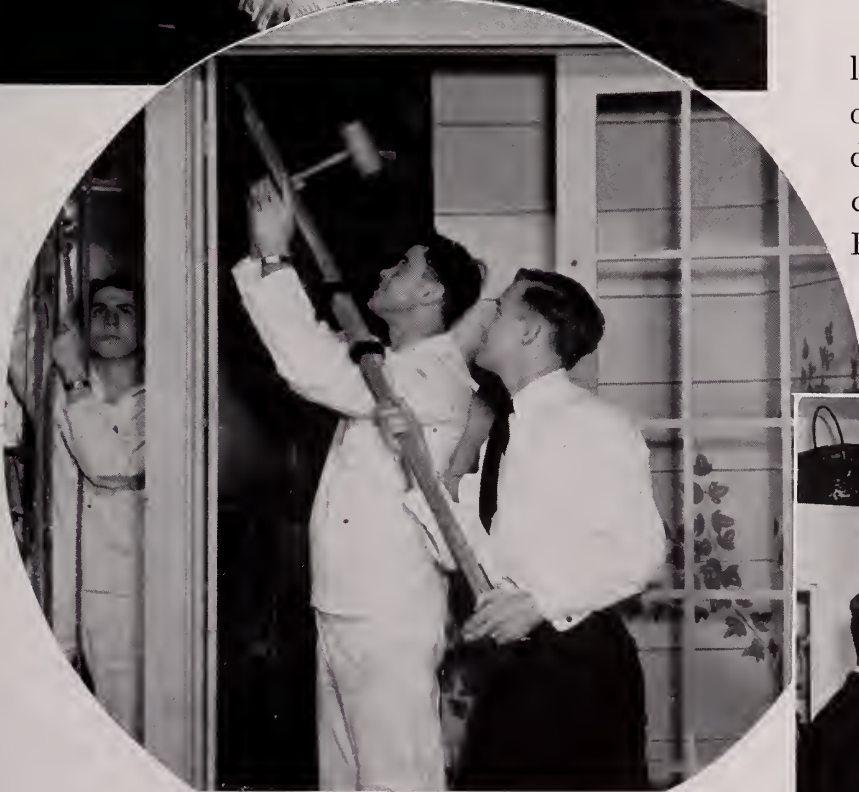
Play house construction engineers
